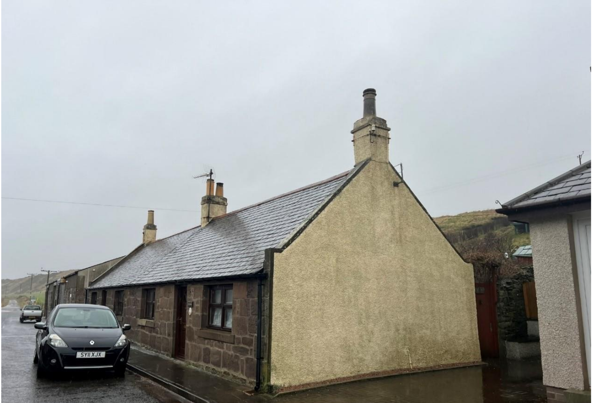
South/Front Elevation, West Street Photo taken 21/02/2024
