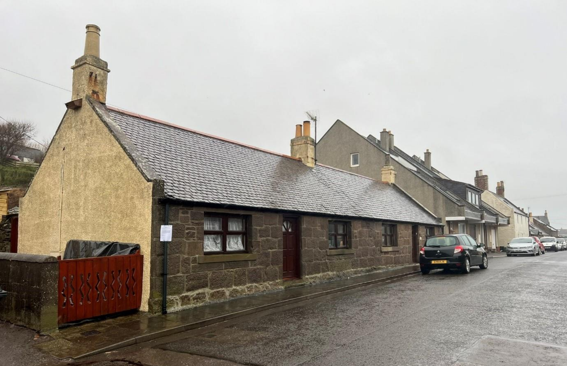
South/front elevation, West Street Photo taken 21/02/2024
