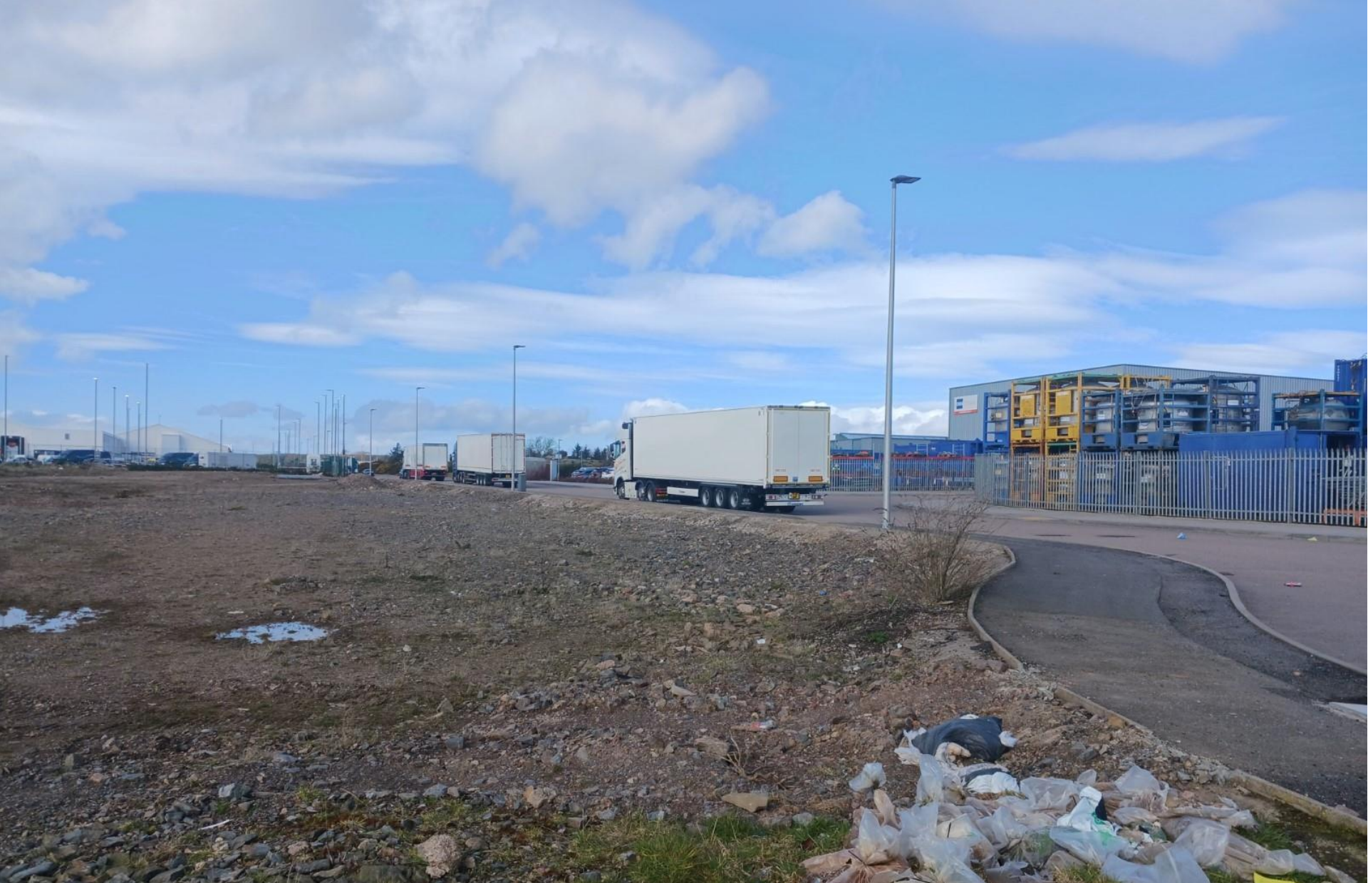
Looking towards the existing warehouse from turning circle from where access to the van storage area would be taken Photo taken 08/04/2024
