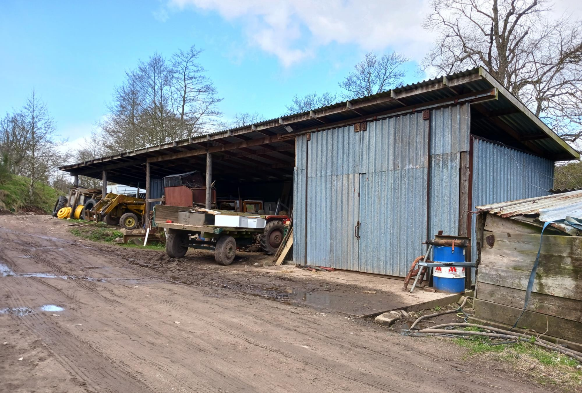
Building located immediately opposite the application site Photo taken 17/04/2024
