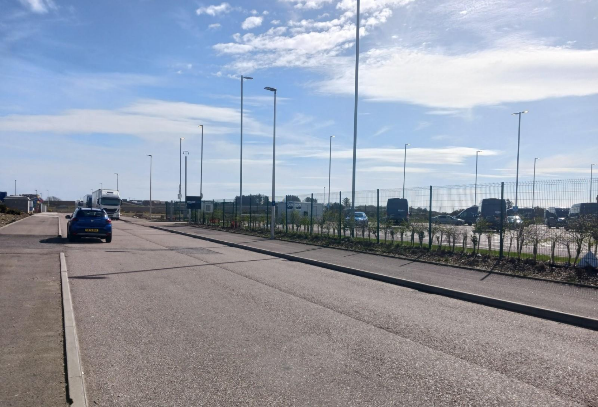
Looking East along Cairnrobin Way Photo taken 08/04/2024
